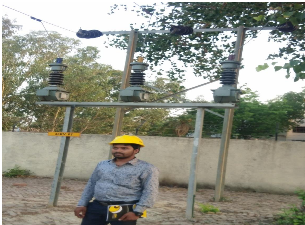
Fig 8: Potential transformer
