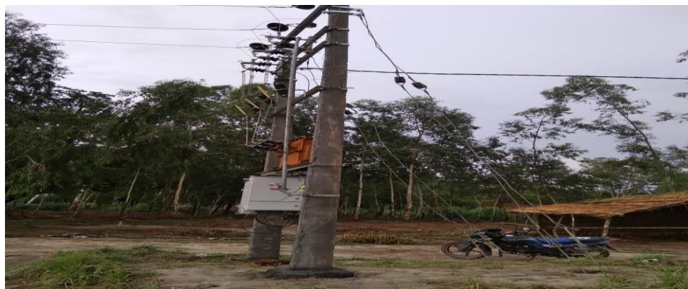
Fig 12: Distribution transformer
